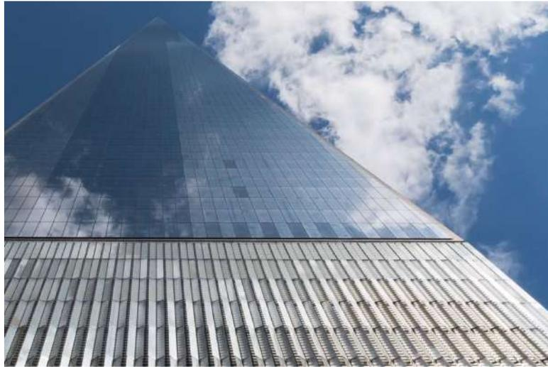
*Figure 8: Example of a Curtain Wall System (Source: Shapiro, G. Architect Magazine)*
